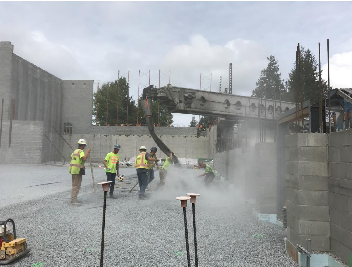
Capillary Break (gravel) Below Future Slab
